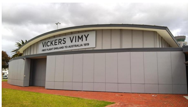
AAL’s interim refurbishment of the Vimy Memorial completed in 2017 [M Milln]
